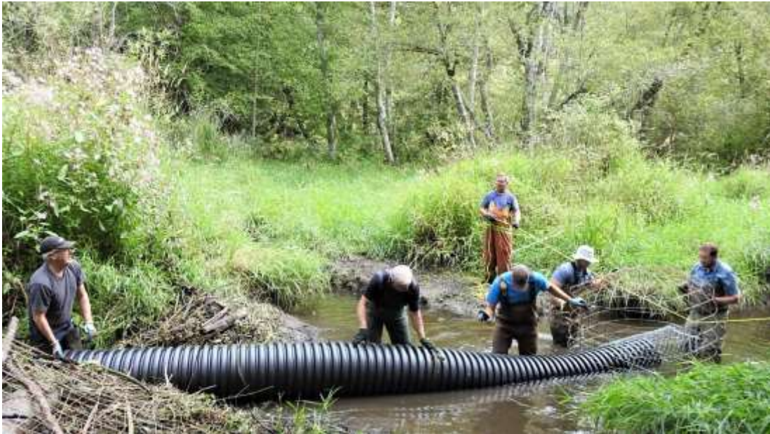
Volunteers and Delta staff install pond leveller through beaver dam in Lower Cougar Creek. Photo Carol Pan More photos at https://drive.google.com/drive/folders/1xZZIC_wL0xIQpKu1cZY-x05uyNU3dd5?usp=sharing
